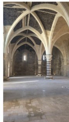
Vaulted stonework inside Castello Maniace.
